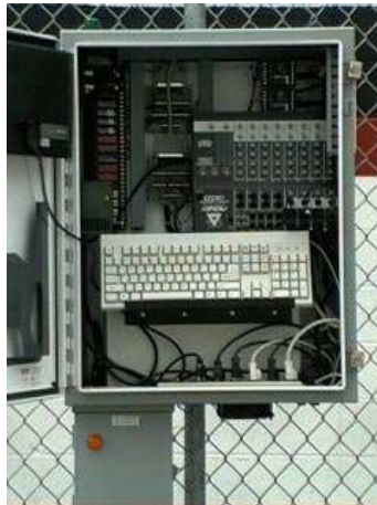
Figura 40. Controlador de nivel de fluido. Fuente: Optimizing pumping well efficiency with smart fluid-level controller technology.
