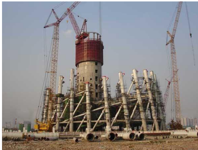
Figura 20. Núcleo en concreto Canton Tower. Tomado de http://www.solaripedia.com/13/342/4264/canton_tower_in_itial_construction.html .
