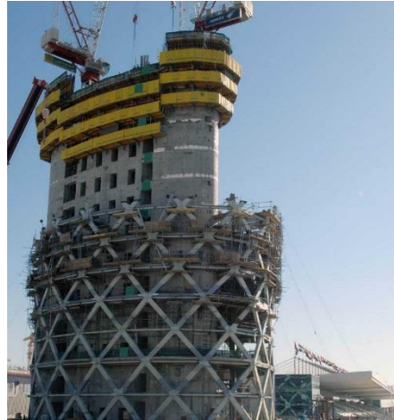
Figura 19. Núcleo en concreto (Capital Gate). Tomado de https://www.e-architect.co.uk/dubai/capital-gate-abu-dhabi .
