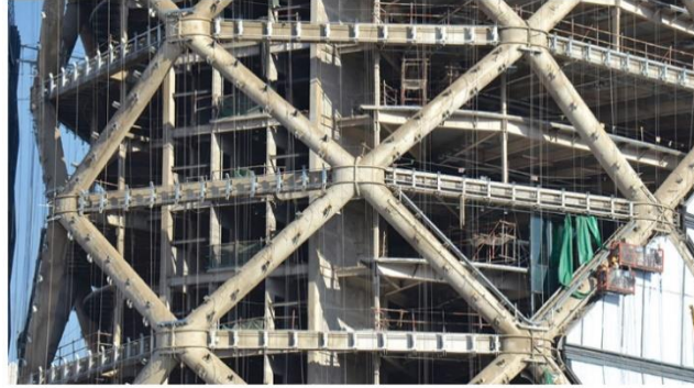
Figura 14. Ángulo poco profundo con respecto a la diagonal. Tomado de https://www.nbmcw.com/tech-articles/tall-construction/38066-unpacking-composite-construction-global-trends.html , 2018
