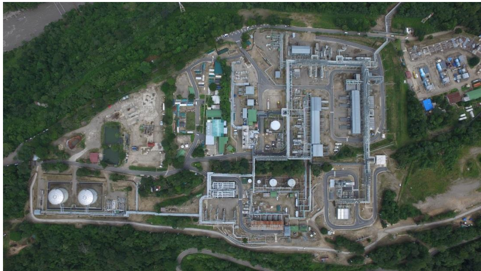
Figura 1. Central Production Facilities Floreña
