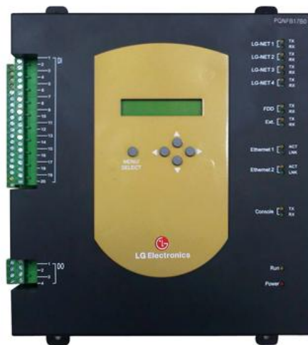
Figura 13. BNU-BACNet (Ref: PQNFB17B0 LG).
