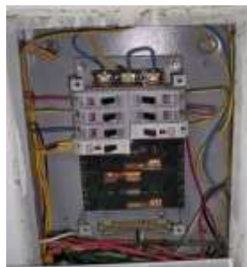
Figura 22 Barraje Tablero TH
