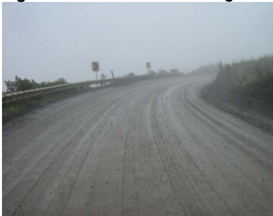
Figura 123. Extendida material granular
