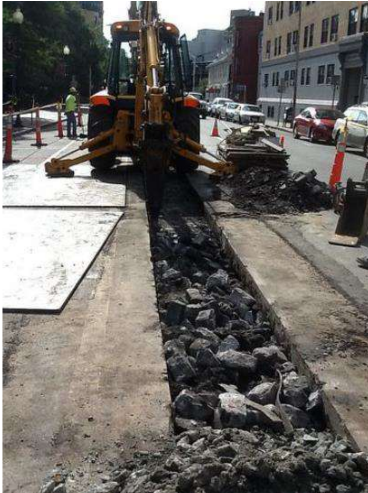
Figura 24. Obras civiles necesarias para soterrar las redes eléctricas. Fuente de la figura: Massachusetts Department of Energy Resources, FEASIBILITY STUDY FOR UNDERGROUNDING ELECTRIC DISTRIBUTION LINES IN MASSACHUSETTS, 2014 (Massachusetts Department of Energy Resources, 2014)
