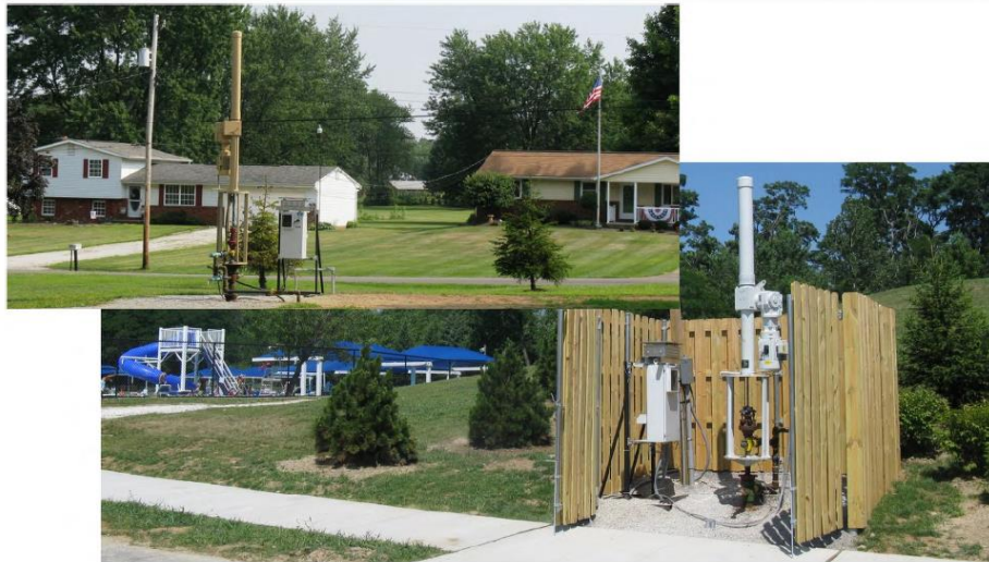
Fuente: Unico Inc. Drives and Systems. Installation records 2009
