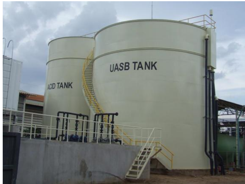
Figura 19. Reactor UASB
