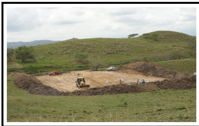
Figura 23: Desmonte y descapote
