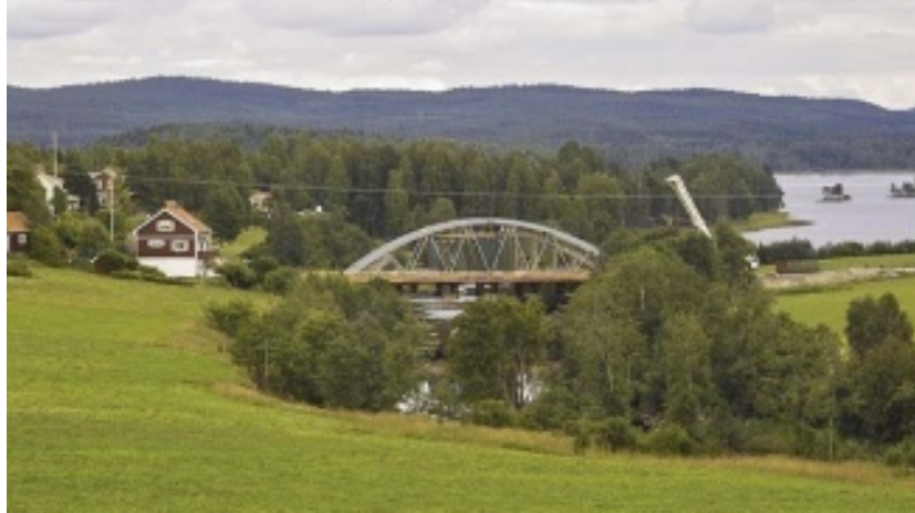
Figura 53. Puente integral OverHokviksan
