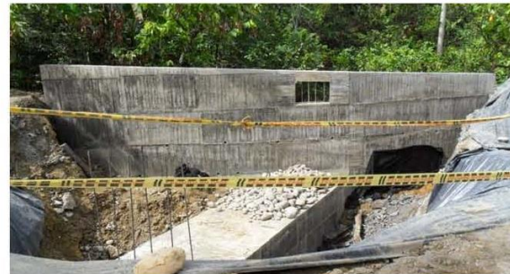
Foto No 2. RELLENO BOX CULVERT K40+620.
