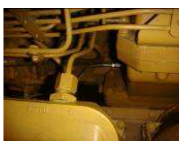
Figura 28 Termoc Manifold Air
