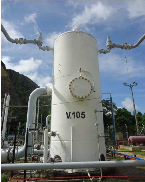
Figura 5 Scrubber V-105 descarga de compresor C-108
