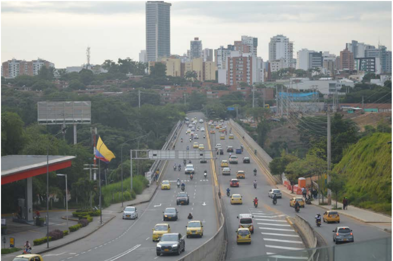
Figure 4. Case study: “La Flora” bridge.
