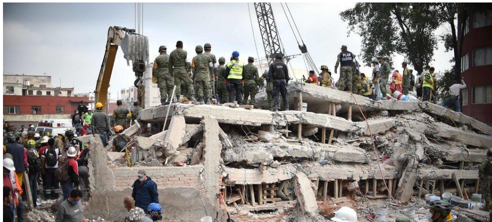
Figura 10. Edificio colapsado México (The New York Times, 2017).
