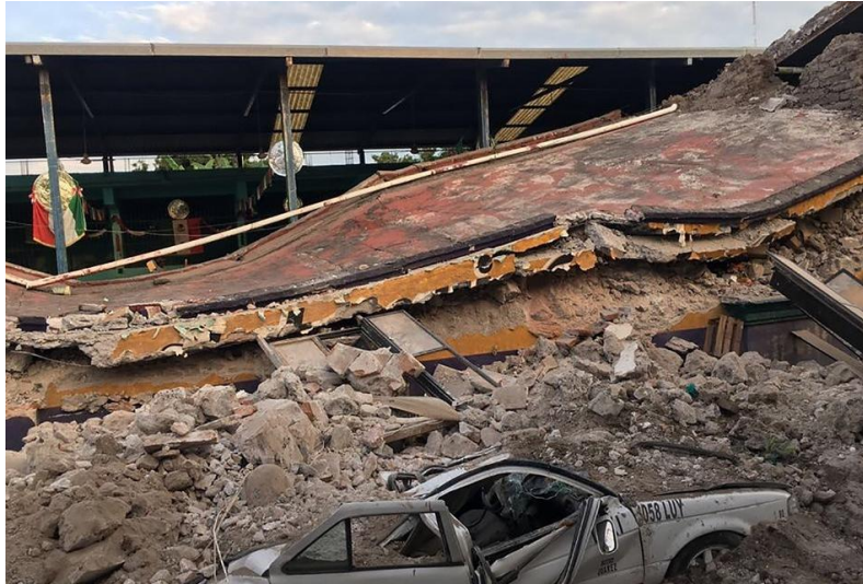
Figura 9. casa colapsada (The New York Times, 2017).
