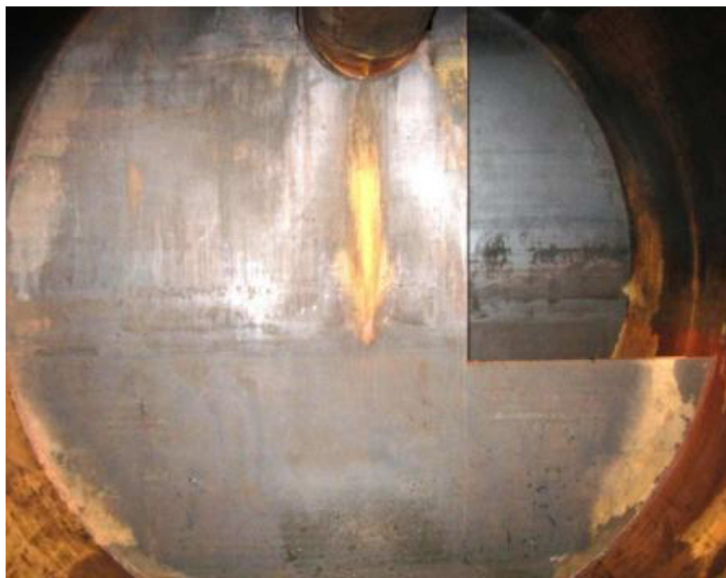
Figura 17. Limpieza surge drum URG 1.
