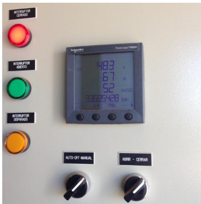
Figura 11. PM810 Power Logic
