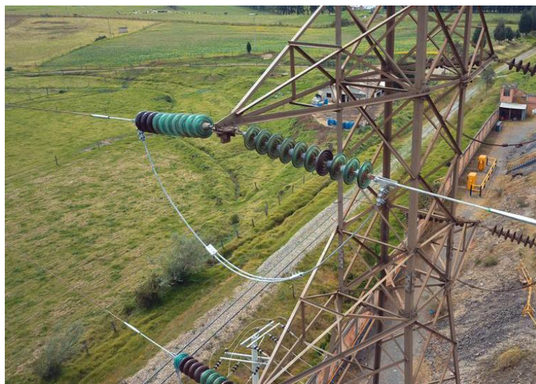
Figura 14. Conductor ACSR 336.4 LINNET
