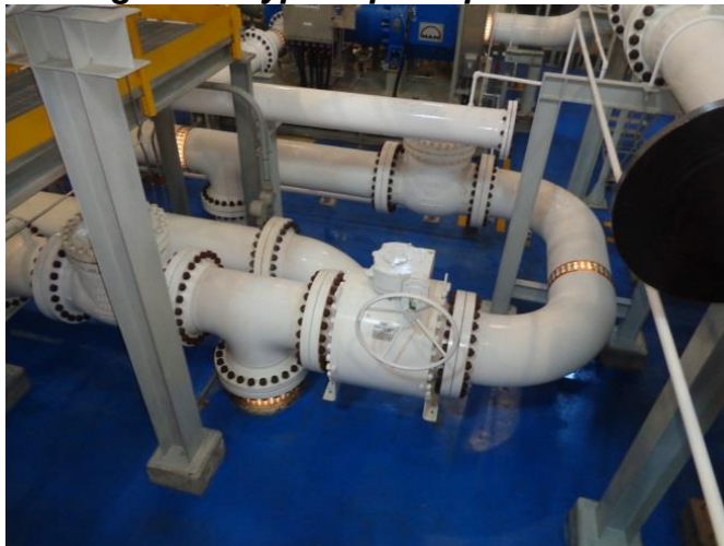
Figura 3. Bypass principal ECGSB.
