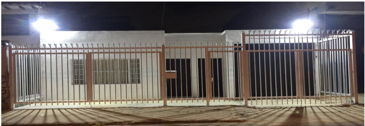
Figura 3. Fachada instalaciones Hydrostatic Testing S.A.S
