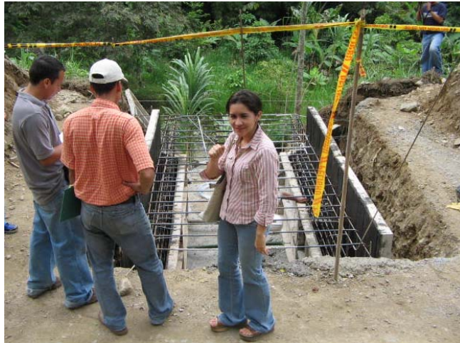
Figura No. 19 Box-Culvert 1.5X1.5
