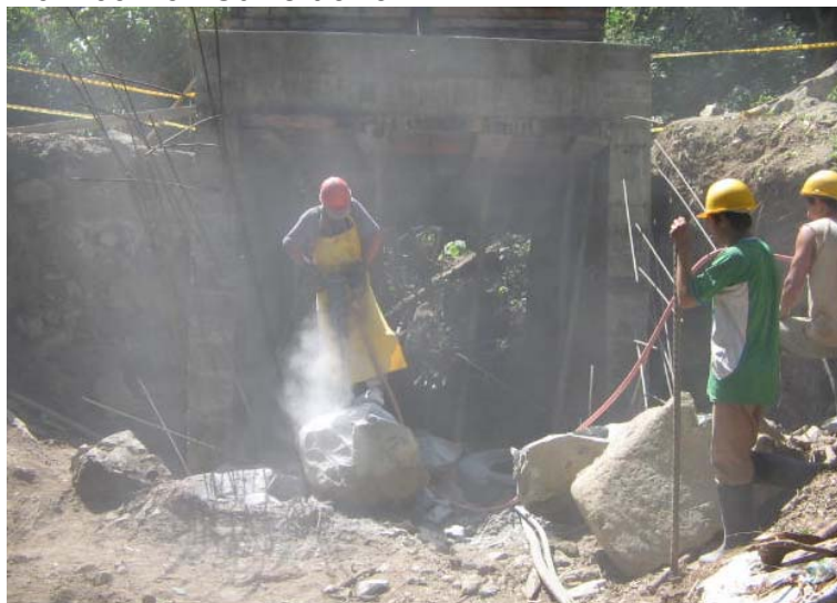
Figura No. 20 K6+709 Box-Culvert 3X3
