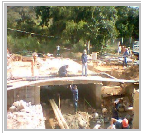
Canal cerrado (Box-Culvert)
