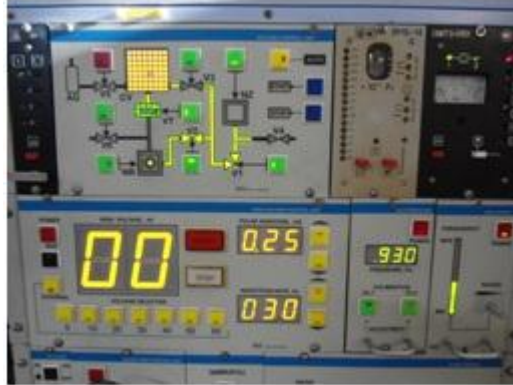
Figura 6. Panel de control del reactor MOSMET
