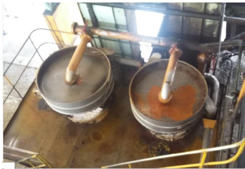
Figura 27. Tamices extractora central
