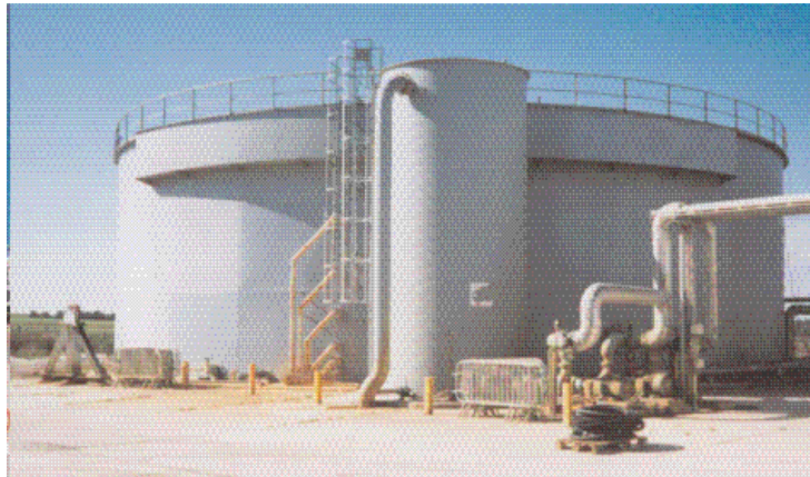
Figura 5 Reactor UASB a escala industrial
