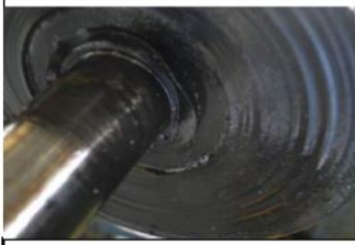
Thrust runner was found with severe wear
