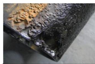
Housings surface presented possible corrosion
