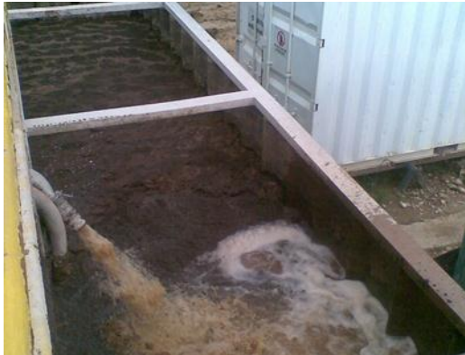
Figura 60. Agua residual industrial
