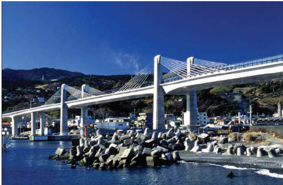
Extradosed bridges in Japan, Akio Kasuga
