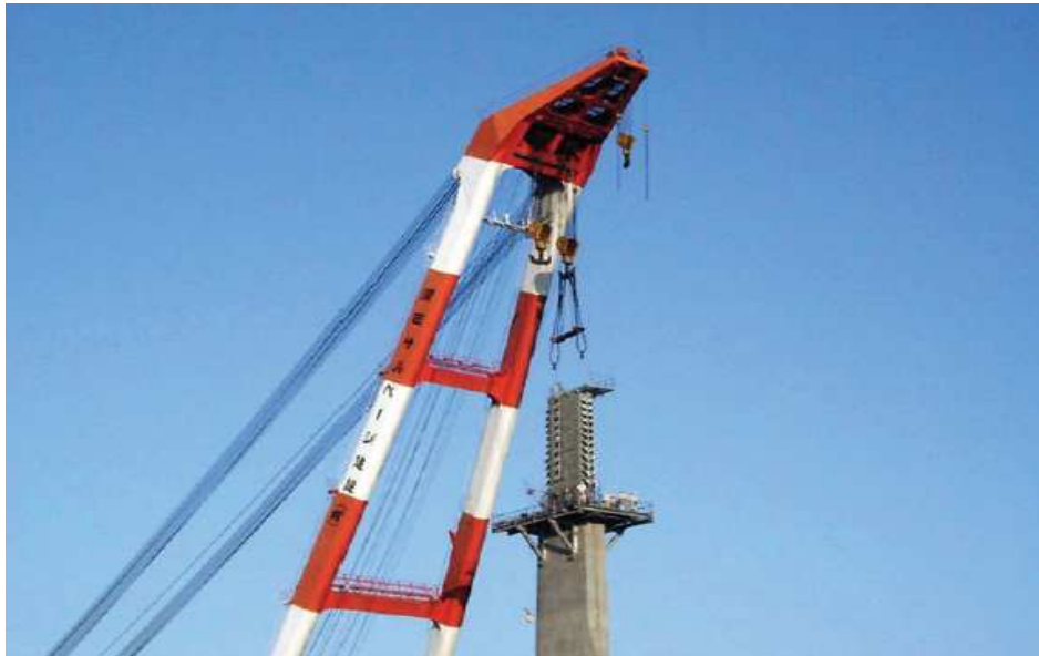
Extradosed bridges in Japan, Akio Kasuga
