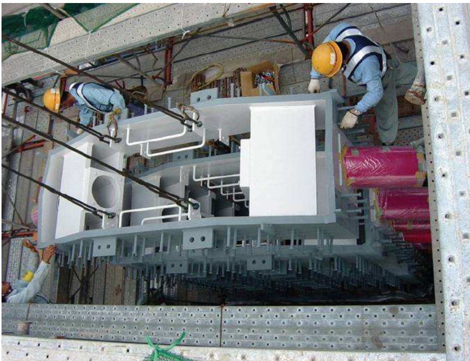
Extradosed bridges in Japan, Akio Kasuga
