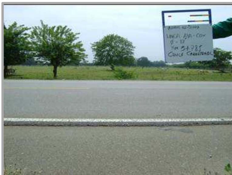
Figura 23. Cruce carreteables principales, Km 3+785.
