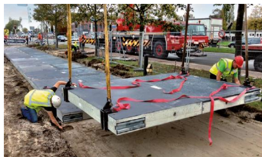
Figura 21. Carril para bicicletas en Holanda. Adaptada de SOLAROAD, “Paving the way to the road of the future, pdf
