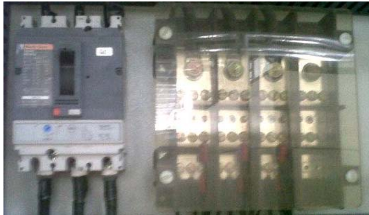
Figura 16. Bornera e interruptor Compact NS Merlin Gerin- 3 polos, Compact NS100N TM100D 100A/40°C MERLIN GERIN
