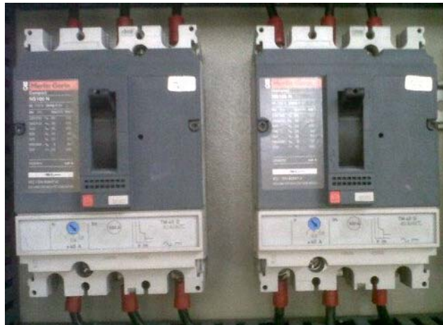
Figura 17. Interruptores Compact NS Merlin Gerin- 3 polos, Compact NS100N TM100D 40A/40°C MERLIN GERIN
