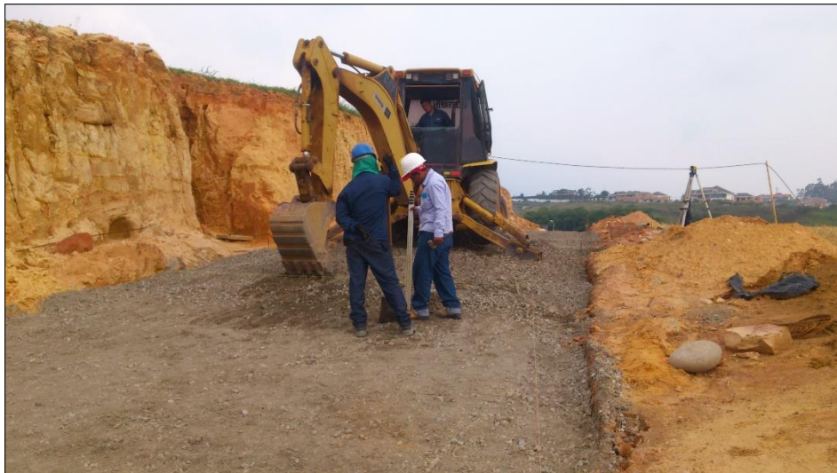
Figura 13. Extendida base granular
