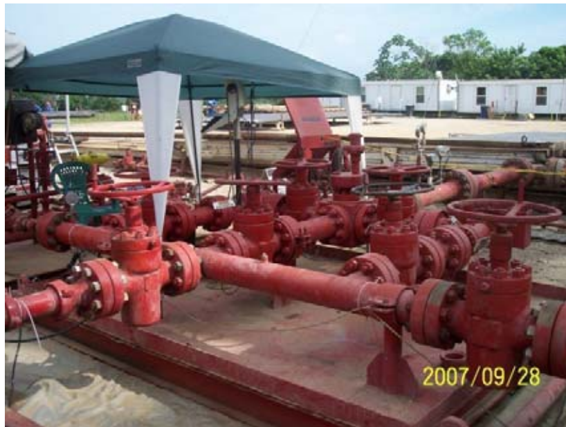
Foto 4-3: Choke Manifold
