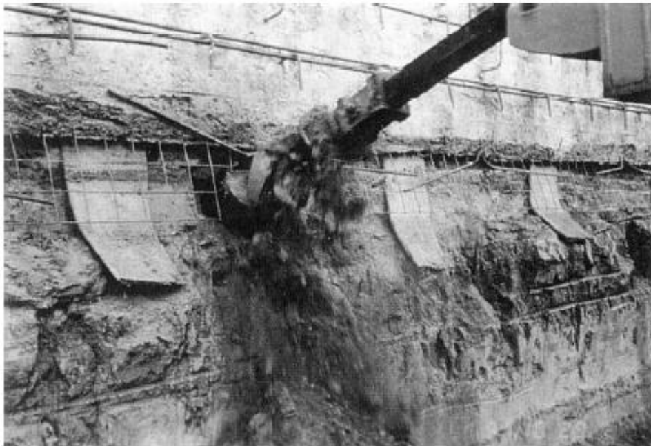
Soil Nail Walls
