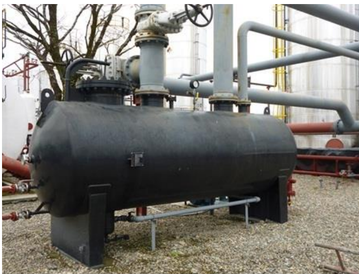
Figura 19. KO Drum y Scrubber
