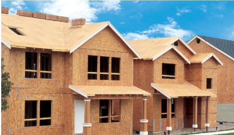
Figura 31. Tableros de madera contrachapada (*The Engineered Wood Association APA., 1997*)
